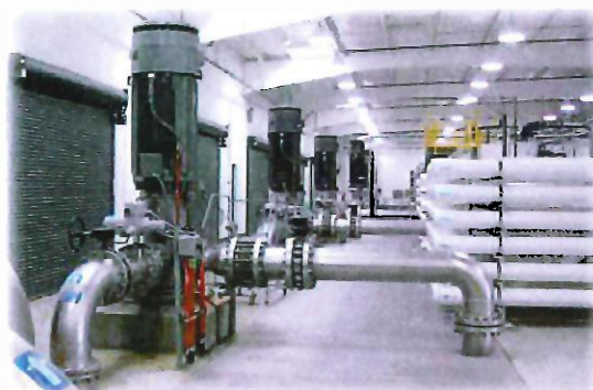
Chino II Desalter Treatment Facility
