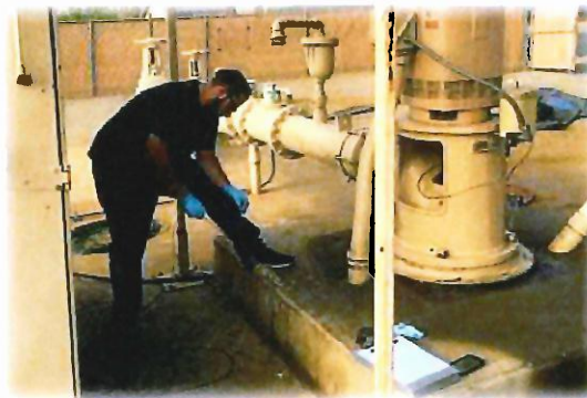
Maintaining Transducer Equipment in One of the Well Sites
